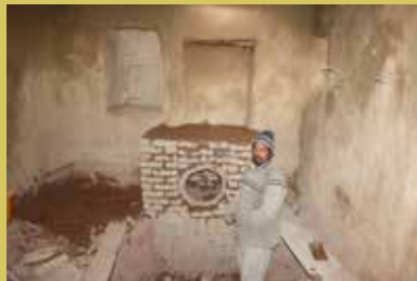
Tandoor installed for testing
